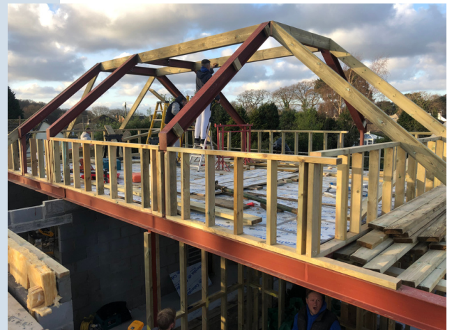
New roof joist being fitted
